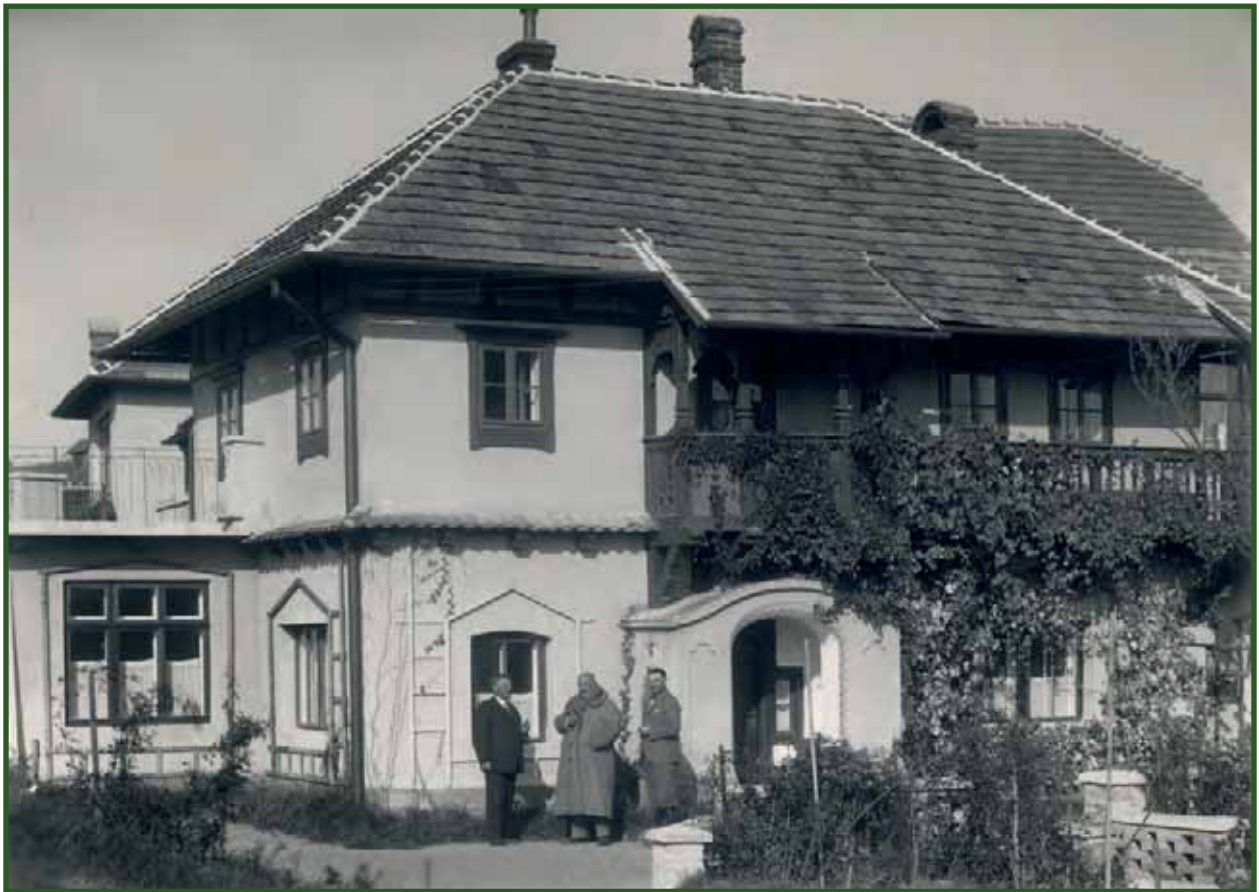
The villa in Hroznova Lhota in the early 20 th century after the restoration by architect, Dusan Jurkovic.
